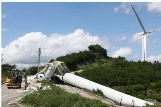
By typhoon damaged wind turbine in September 2020 https://en.yna.co.kr/view/PYH20200903214900325 (25.02.2021)
