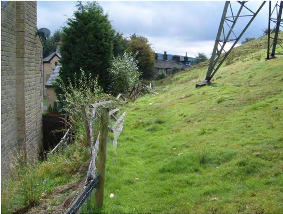
Plate 4 Tower on Unstable Slope
