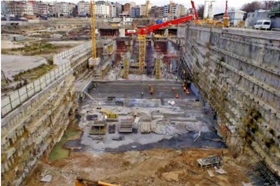
**3.1.5 Yenikapı Ventilation Building: Secant piles + steel struts**
