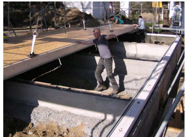
illus. 2 erecting of wooden floor plate over concrete foundation
