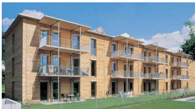
Multifamily house Ölbündt, Dornbirn, Vorarlberg, Austria.
