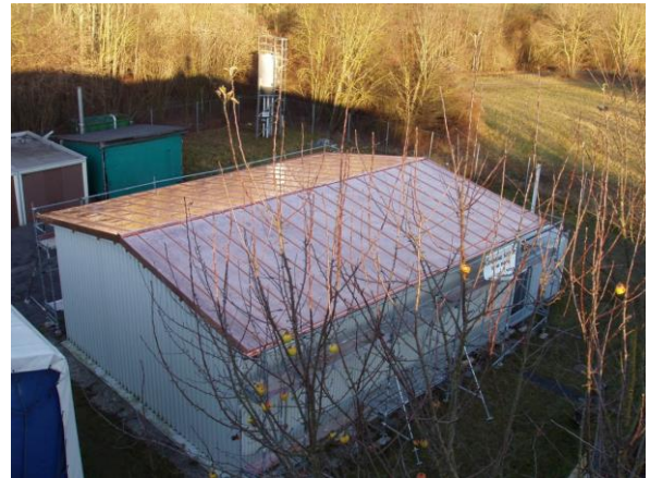
Figure 20: Copper roof runoff for testing treatment plants
