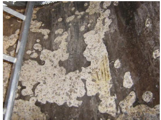
Figure 25: Concrete corrosion within a digester headspace © Rolf König
