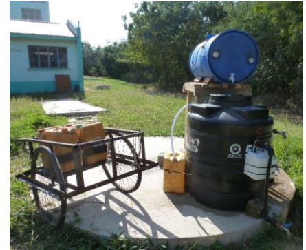
Figure 37: Sandfilter for treatment of river water (Foto: Tim Fettback / Nils Horstmeyer)
