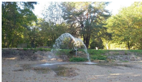
Figure 29: Infiltration basin on the island Baumwerder, Lake Tegel
