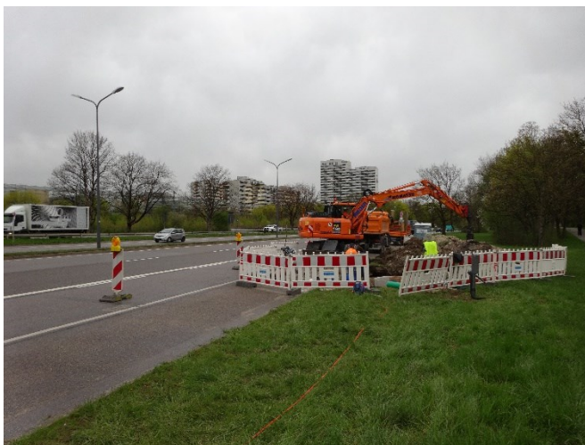
Figure 16: Installation of a decentralized treatment plant for road runoff
