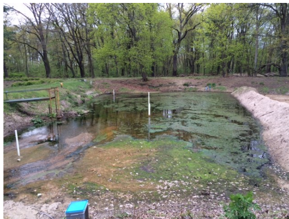
Figure 24. Infiltration basin on the island Baumwerder, Lake Tegel
