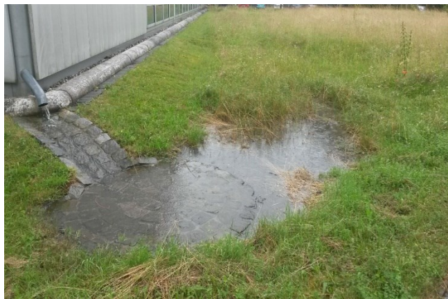
Figure 17: Vegetated infiltration swale at a zinc roof
