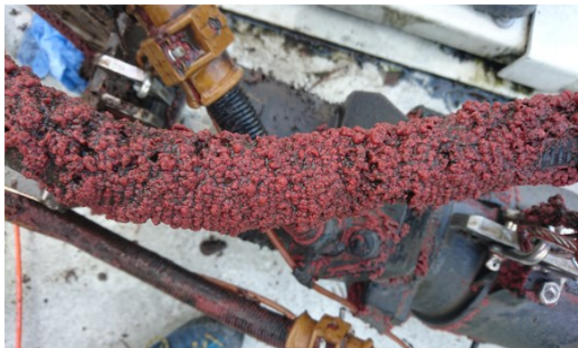
Fig. 2: Deammonifying biomass inside the SBR.
