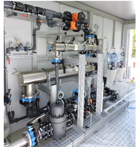
Fig. 39: UV/H 2 O 2 pilot plant at WWTP Gut Marienhof (Munich II).
