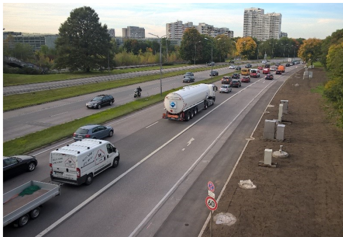
Fig. 21: Testing facility for traffic area runoff treatment.
