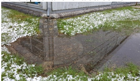
Fig. 5: Vegetated infiltration swale treating zinc roof runoff
