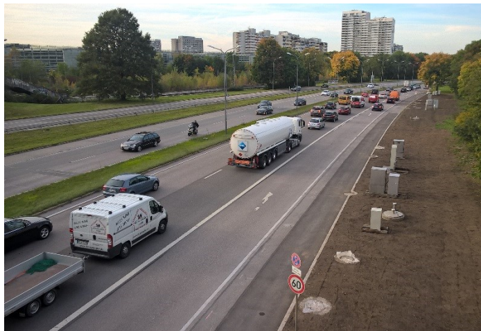
Fig. 7: Testing facility for traffic area runoff treatment
