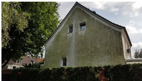
Fig. 9: Biocides inhibit unwanted organisms on building facades
