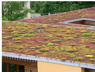
Figure 4: Example for an extensive green roof. Photo: Brigitte Helmreich
