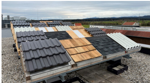
Figure 8: Construction of the test roofs in the field
