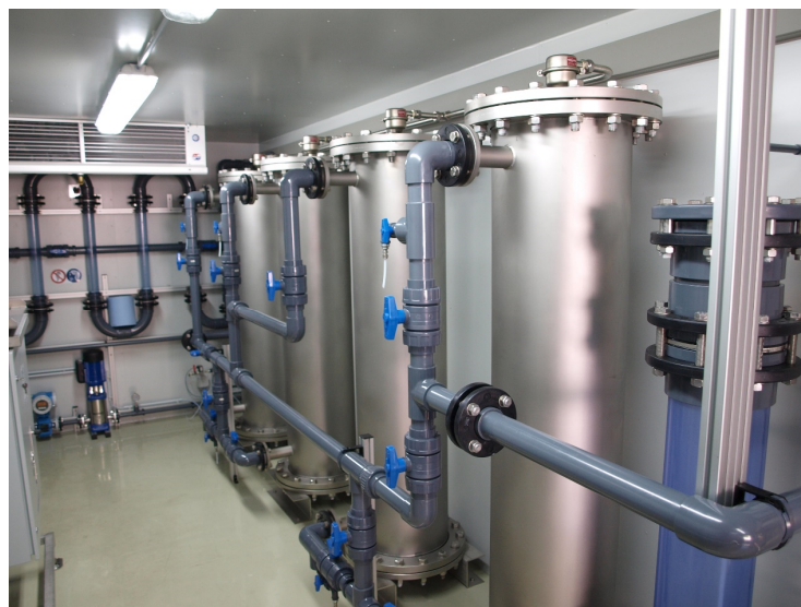
Figure 29: Second barrier in the Nutzwasser treatment train (ozonation).
