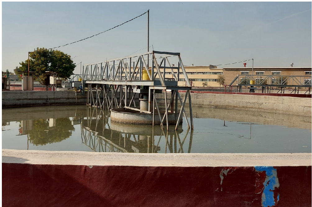
Figure 43: A primary clarifier in a wastewater treatment plant in Tashkent, Uzbekistan.
