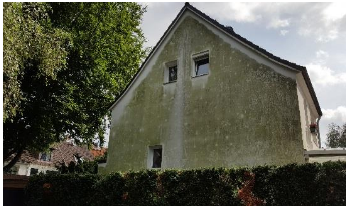
Figure 10: Biocides inhibit unwanted organisms on building facades
