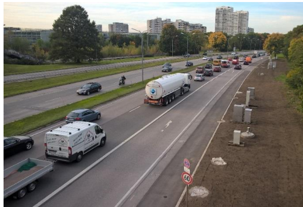
Figure 9: Testing facility for traffic area runoff treatment
