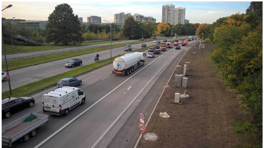
Figure 7: Testing facility for traffic area runoff treatment.
