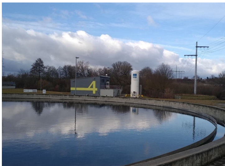
Figure 38: Advanced treatment unit at the wastewater treatment plant Weißenburg.
