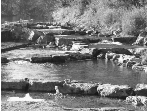
Fig. 4.7.20(a): Overview of the fish ramp Leitner at low flow condition
