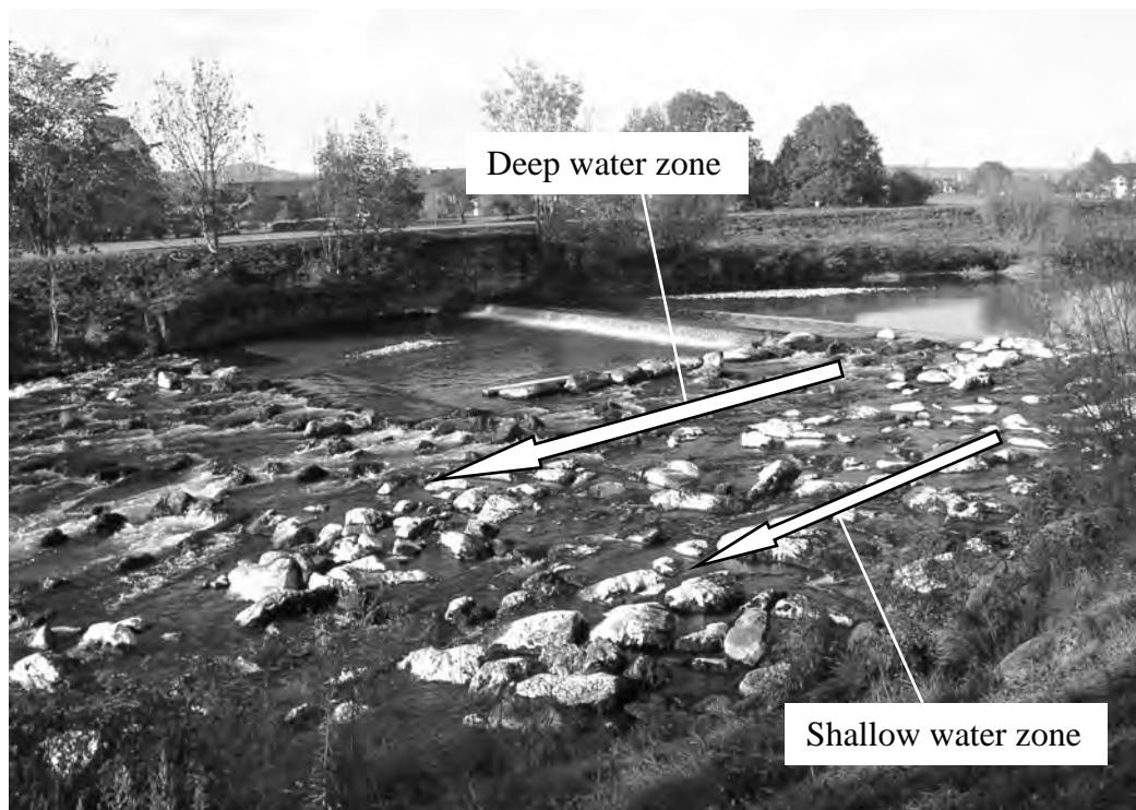
Fig. 4.5.4(a): Fish ramp Schwaig in the river Mangfall, photo made on Oct.26.2006, Q = 4.84 \text{ m}^3/\text{s} (correspond to Q_{30} )
