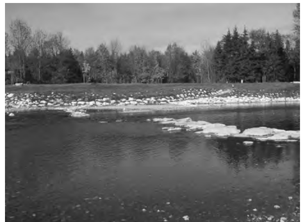
Fig. 4.4.21(f): View of the resting pool and the boulder sill.
