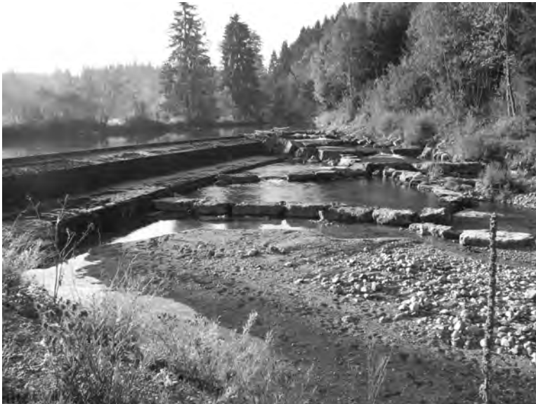
Fig. 4.7.5: Fish ramp Leitner Mühle, photo made on Oct.12.2006, Q = 3.09 \text{ m}^3/\text{s} ( \approx Q_{30} )
