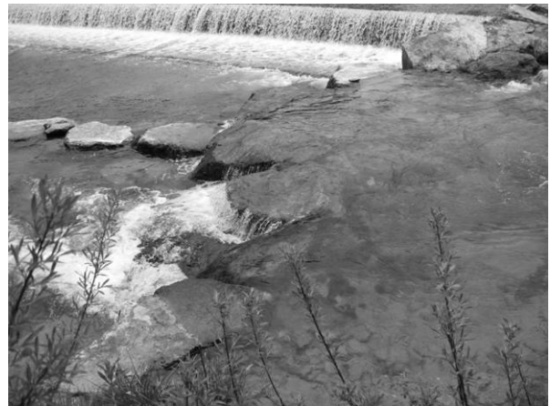
Fig. 4.7.10(d): Boulder sill No. 5, the drop height here is about 34 cm.
