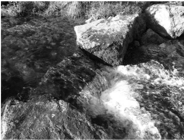
Fig. 4.7.20(c): Boulder sill No. 5, drop height was about 39 cm
