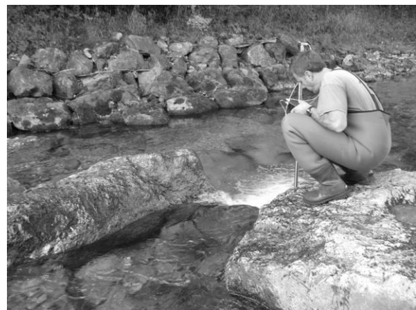
Fig. 4.7.20(f): Boulder sill No. 15, drop height was about 43 cm
