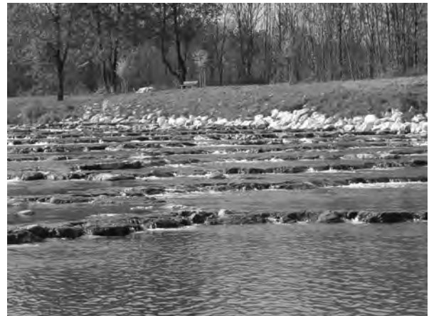
Fig. 4.4.21(d): Close view of the upper ramp from downstream. Seems to be lack of suitable passage
