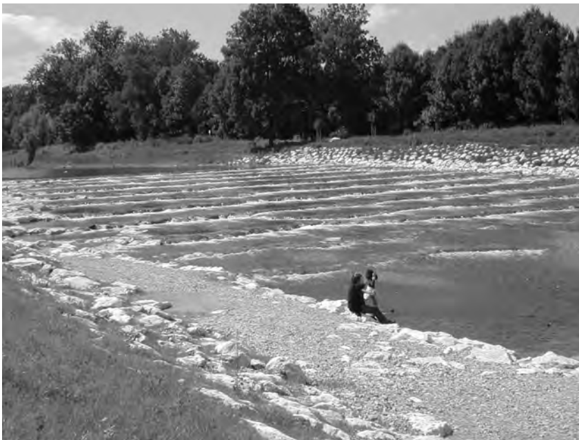
Fig. 4.4.5: Bottom ramp Kolbermoor in the river Mangfall, photo made on Aug.09.2005, Q = 39 \text{ m}^3/\text{s} ( \approx Q_{330} )
