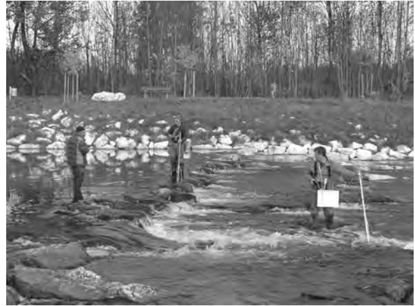
Fig. 4.4.21(b): In the middle at the first boulder sill of upper ramp, flow concentrated well during low flow.
