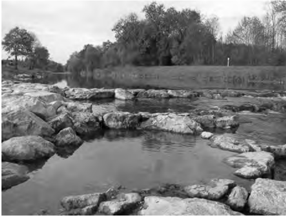
Fig. 4.4.21(a): During low flow condition, no overflow at some parts of the ramp
