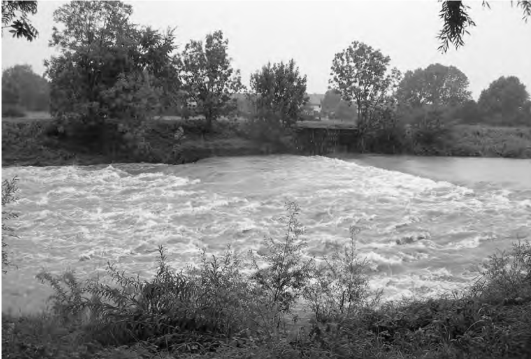
Fig. 4.5.4(b): Fish ramp Schwaig in the river Mangfall, photo made on Sep.03.2007, Q = 56.4 \text{ m}^3/\text{s} (correspond to 1.5 \times Q_{330} )
