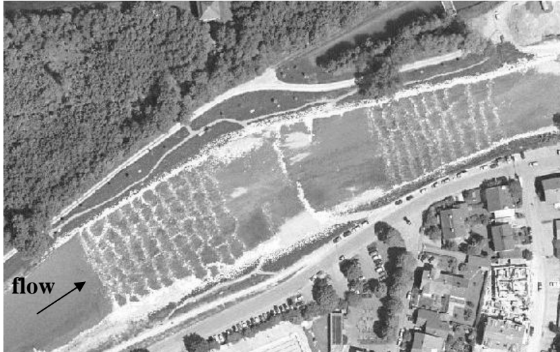
Fig 4.4.4: Bird's eye view of the bottom ramp Kolbermoor
