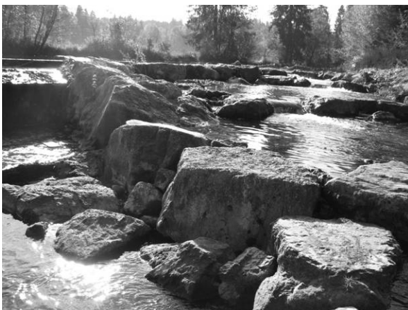
Fig. 4.7.20(e): Inserted amourstones
