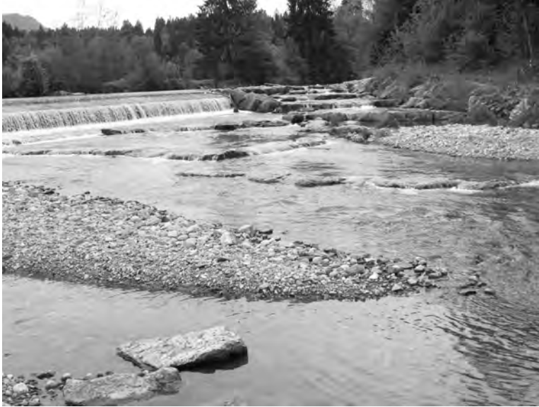
Fig. 4.7.4: Fish ramp Leitner Mühle, photo made on May.23.2006, Q = 6.10 \text{ m}^3/\text{s} ( \approx \text{MQ} )
