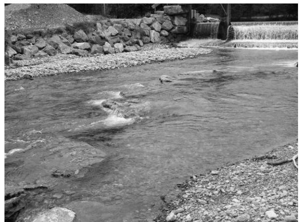
Fig. 4.7.10(f): Boulder sill No. 13
