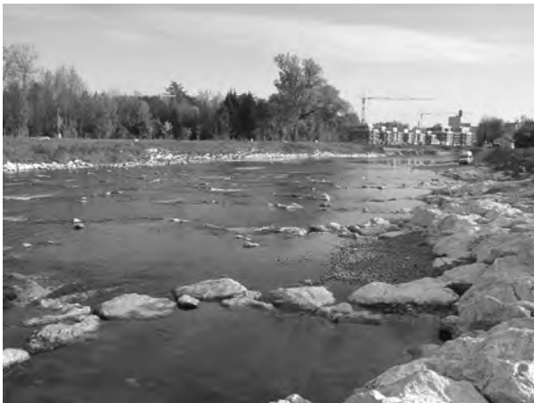
Fig. 4.4.21(c): View of the upper ramp from upstream
