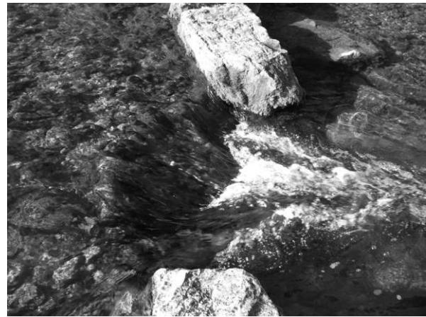
Fig. 4.7.20(d): Boulder sill No. 8, drop height was about 19 cm
