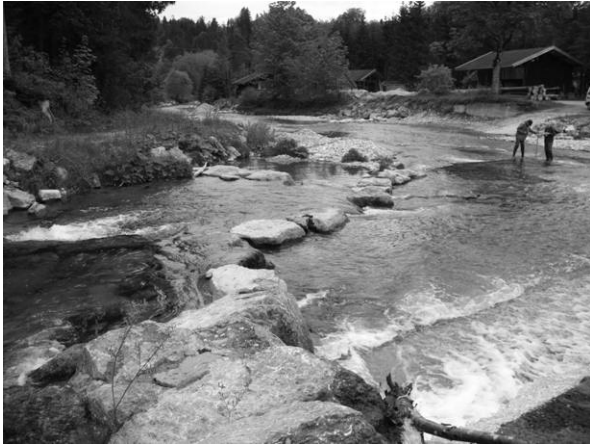
Fig. 4.7.10(a): Overview of the fish ramp Leitner
