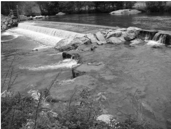
Fig. 4.7.10(c): Boulder sill No. 4, the drop height here is about 30 cm
