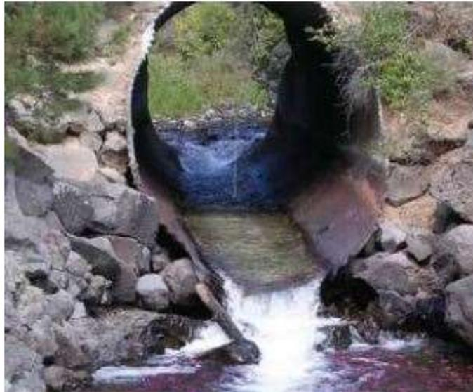
**Figure 2.2:** Culvert fishway (Forest Service Stream-Simulation Working Group, 2008).
