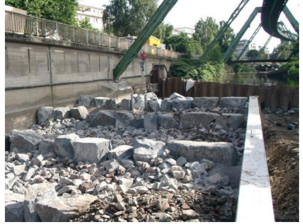
Figure 1: Example cross-bar block ramp under construction (source: Wupperverband)
