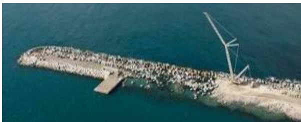
Figure 17. Breakwater state after the 15/2/11 storm. Overview and details
