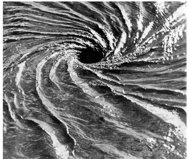
Figure 1: The intake vortex turns clockwise during the emptying through the diversion tunnel (diameter = 7.6 m) at Lake Arapuni (New Zealand). The tunnel submergence was about 21 m (Ball, 1933).
