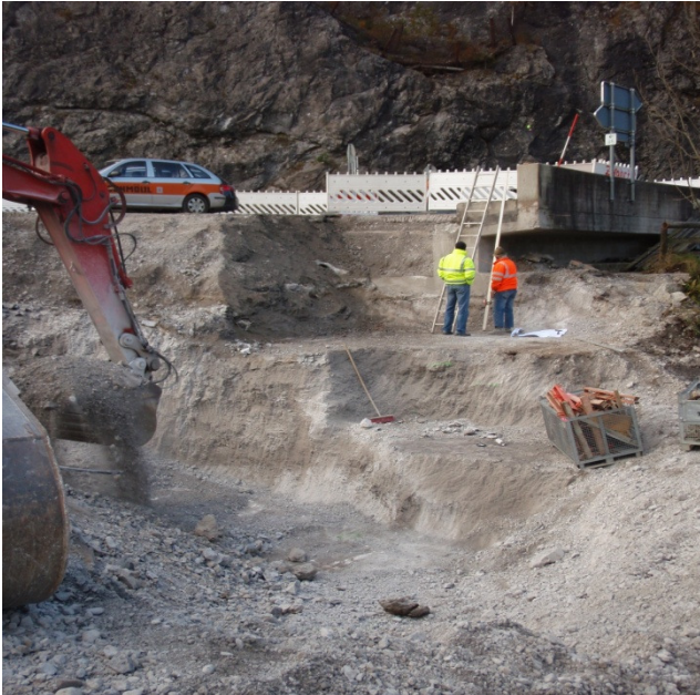
Figure 9: Exposing of the bedrock surface on the Hennenköpfl
