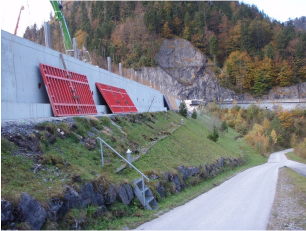
Figure 6: Finished cantilever retaining wall on the air side
