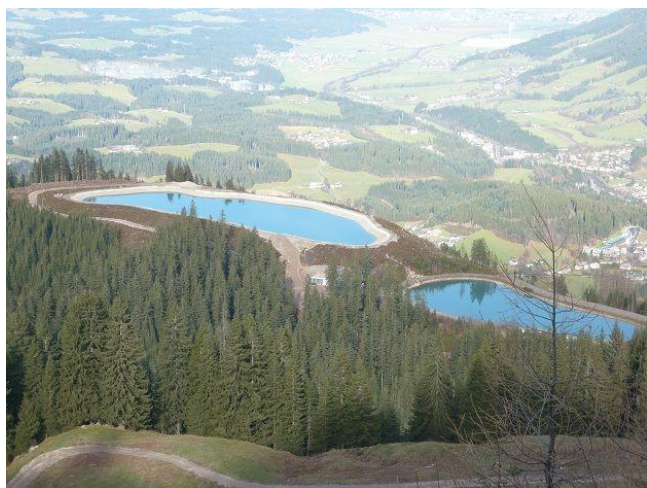
Figure 2: Reservoirs used for the production of artificial snow in the Austrian Alps could be used as small scale pump storage plants (photo from: Hydrosnow, 2010).
