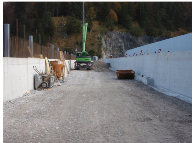
Figure 5: Widening of the dam crest; view looking towards the Sylvenstein cliff
