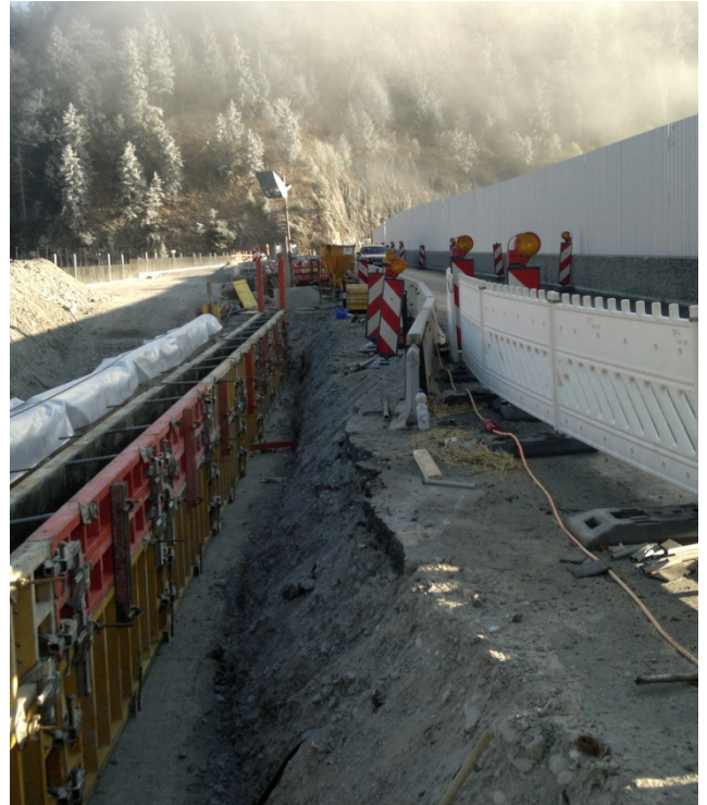
Figure 8: Construction of the training wall
